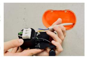
Re-insert the installation disc with the three screws Step 7
